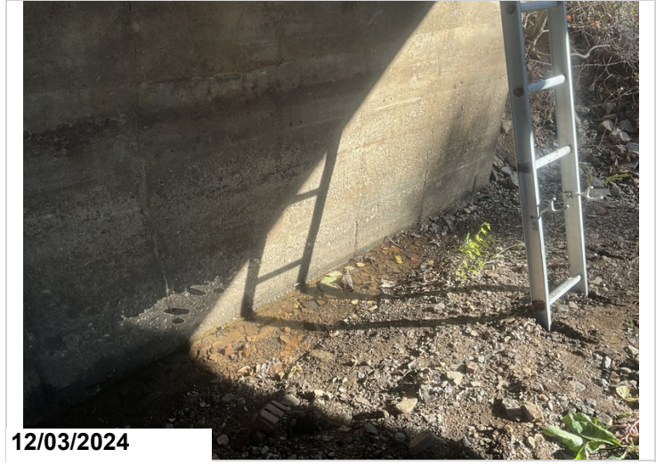
Abutment # 2: exposed reinforcing steel.
