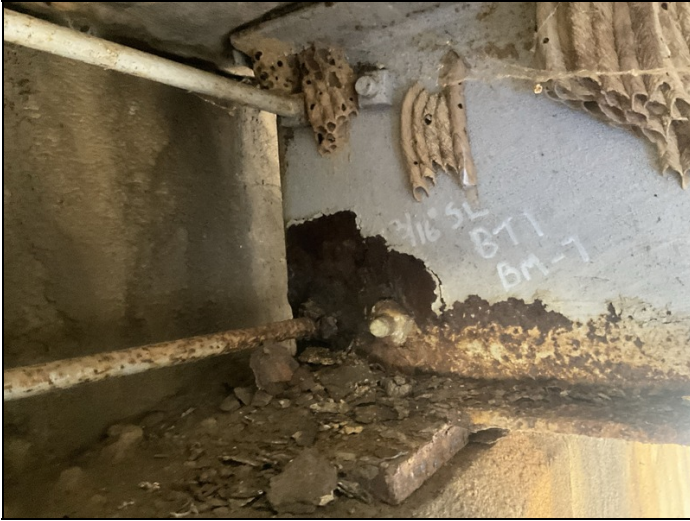
Girders 5, 7, and 12 are the worst having moderate section loss up to 3/16" inch.
