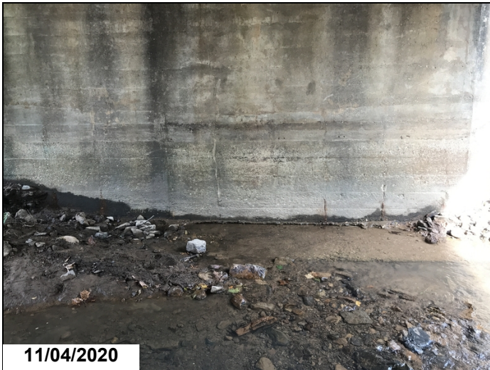
Base of Bent # 2. Exposed reinforcing steel.
