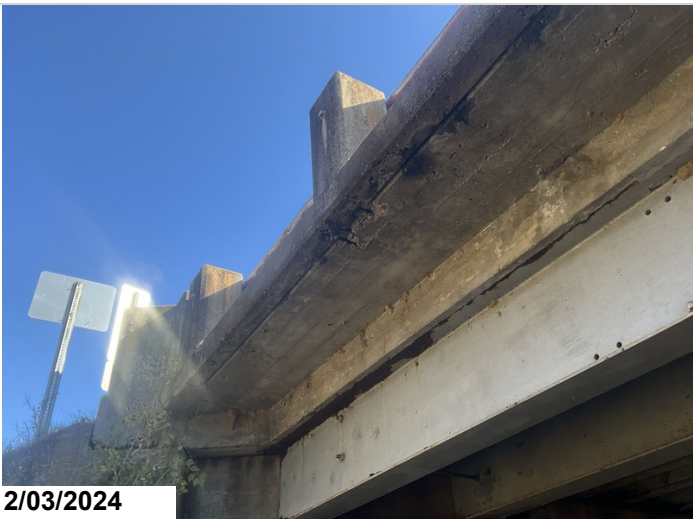
Left overhang spalling with exposed reinforcing steel.
