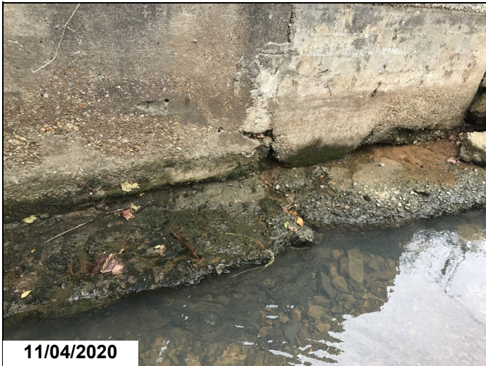
Northwest wing wall and footing concrete deterioration.
