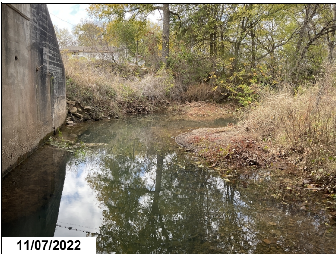
Upstream channel alignment has caused the local scour to pile cap footing at abutment 1.
