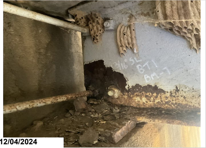
Girders 5, 7, and 12 are the worst having moderate section loss up to 3/16" inch.
