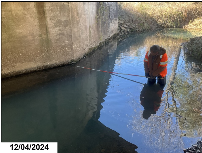
Abutment # 1, left: undermining scale.
