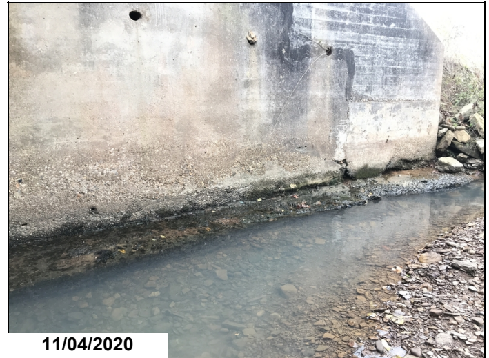
Northwest wing wall. Deteriorated concrete.
