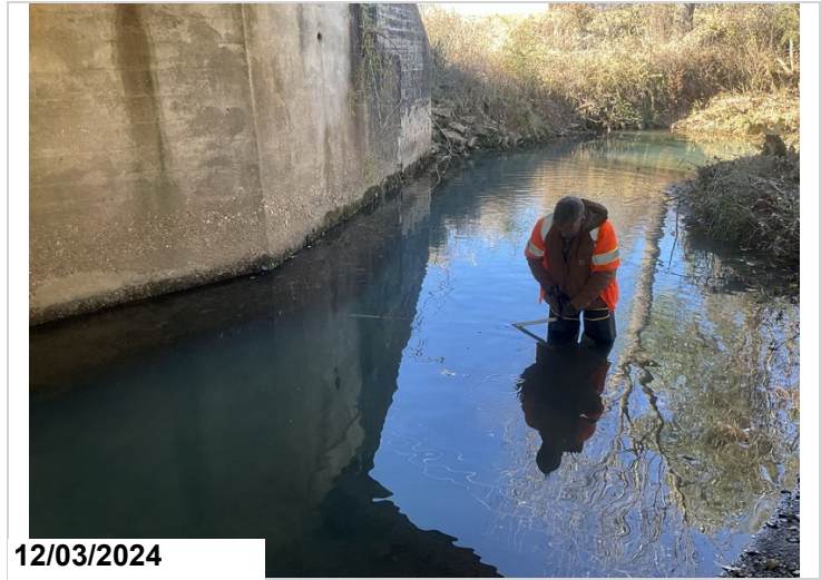
Abutment # 1, left: undermining.
