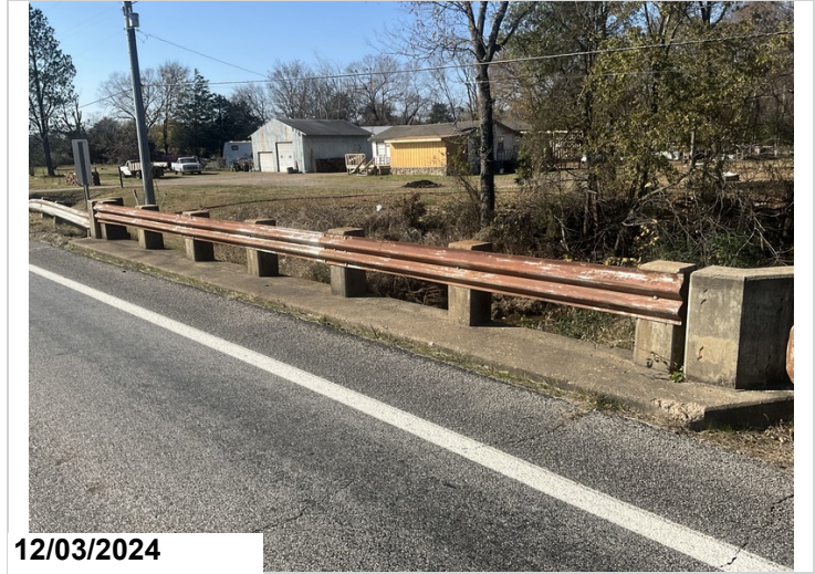
Bridge rail with a failed paint system.
