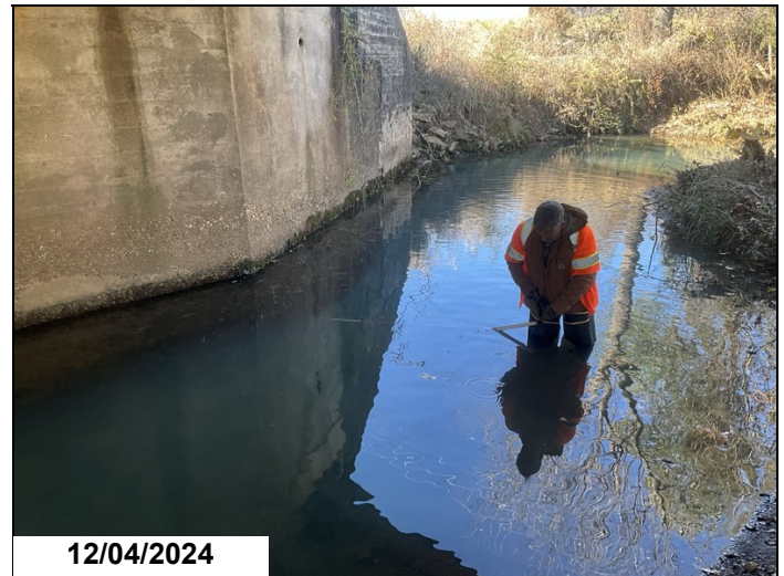
Abutment # 1, left: undermining.
