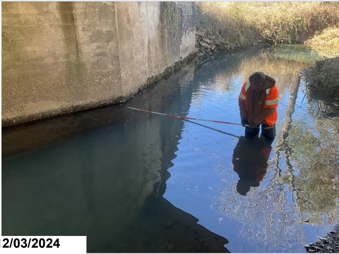
Abutment # 1, left: undermining scale.
