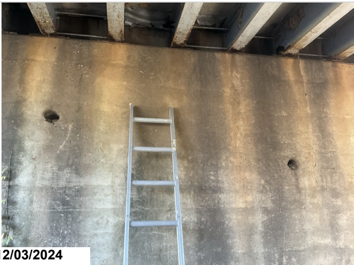
Abutment # 2 moderate width cracking.
