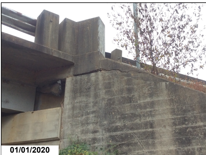
Northwest wing wall has a crack for approximately 4' along the top of the wall.
